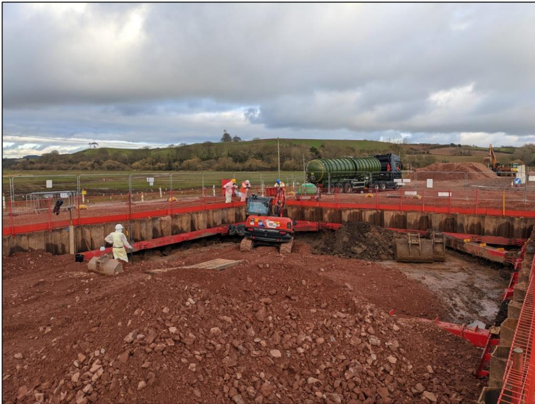
Photo 3. Excavation of contaminated area (Source: Kier)
