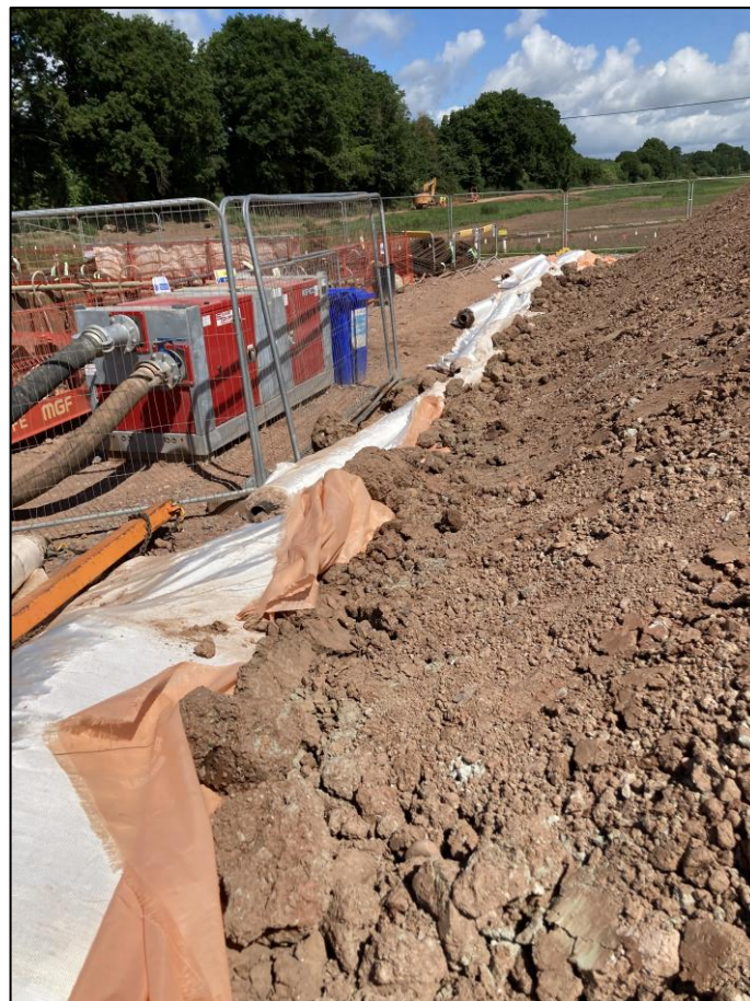
Photo 1. Orange warning geotextile under the new bank (Source: Environment Agency)
