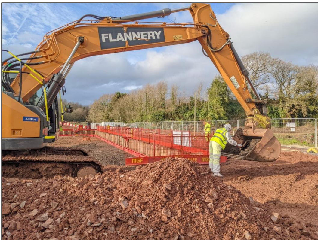
Photo 2. Excavated material controlled for asbestos (Source: Kier)
