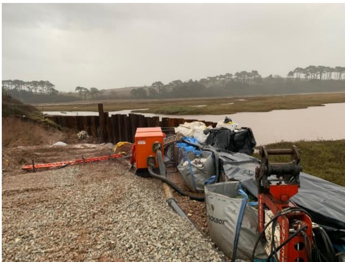
Photo 2.4 Lower Otter embankment being repaired after extensive erosion in 2018 (Source: Environment Agency)
