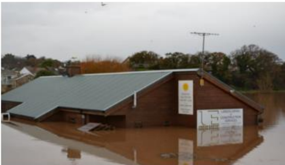
Figure 6.5 BSCC flooded up to its eaves in 2018 floods. Source: Clinton Devon Estates
