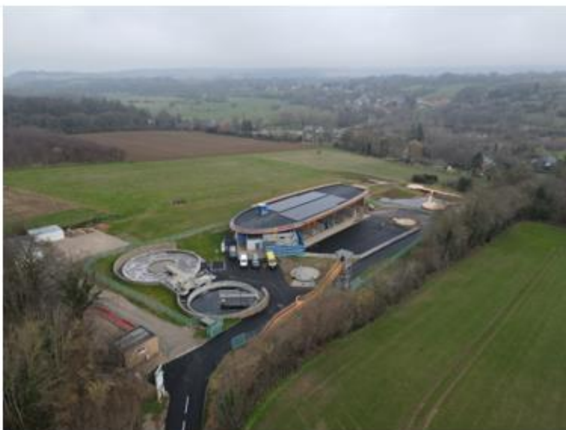
Figure 7.6 New wastewater treatment facility at Longueil. Source: Thomas DROUET/Cdl, 2023
