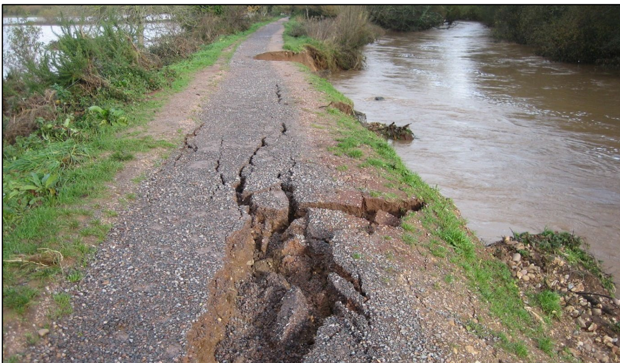
Image 9. Crest level footpath damage caused by flooding in 2012
